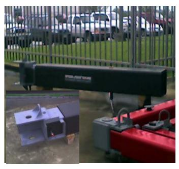
This NEW 10" Manhole Braces is designed to be used as a sheeting and brace type application. The benefit of this system is the hydraulic adjustable 36" inner-sleeve assembly. Used in conjunction with appropriate sheeting, they provide the active support necessary to safely secure excavations.
