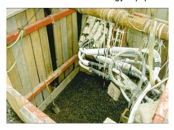
Manhole Braces, used in conjunction with appropriate sheeting provide the active support necessary to secure safe excavations in less stable soils. Available in a wide variety of sizes and capacities, Manhole Braces are composed of modular sections for ease of assembly and transport. Manhole Braces feature 4-way hydraulic support with high-yield telescoping steel sections, and 4-way hose bridles for simultaneous
